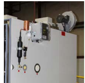
Gas Monitor System
