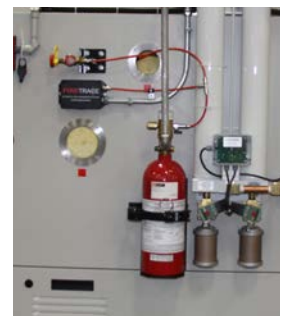
Fire Suppression System
