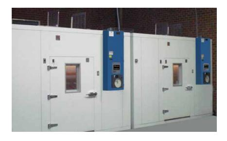
This room is designed to store bottles of pharmaceutical product at -70°C. With over 4800 cu.ft. of conditioned interior space, the chamber is divided into four zones that can each hold up to 288 bottles.
